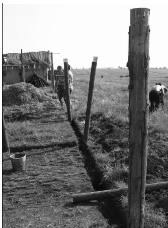
Figure 1. Foundation trenches with wooden posts (Vădastra village, 2005)
