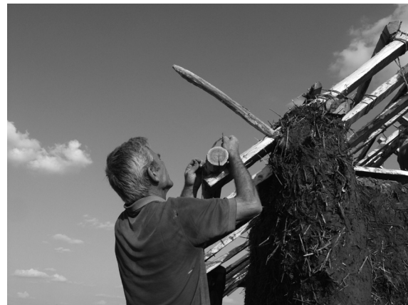
Figure 4. Villager from Vădastra fixing the wooden structure with treads and acacia nails (Vădastra, 2003)
