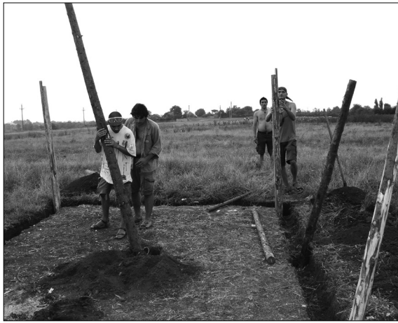
Figure 2. Thrusting into the soil the central post with a movement of rotation (Vădastra village, 2005)
