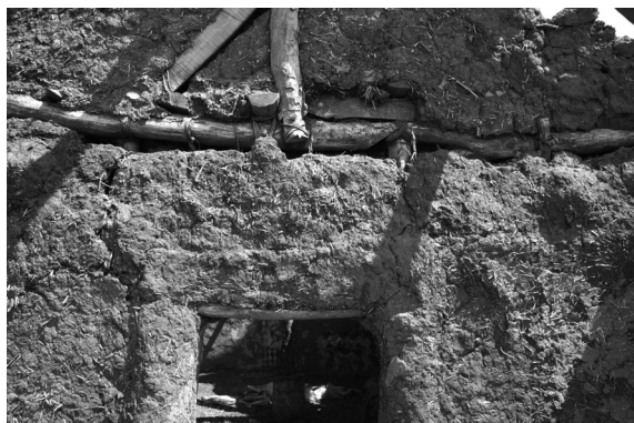
Figure 5. The threads fixtures after a decade of weathering (Vădastra village, 2012)
